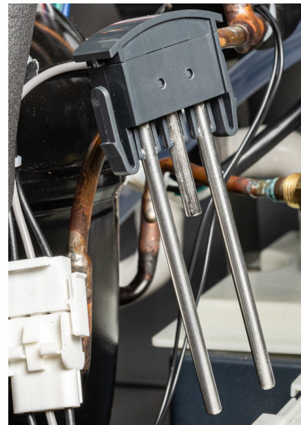
Water Level Sensor A41192-021
